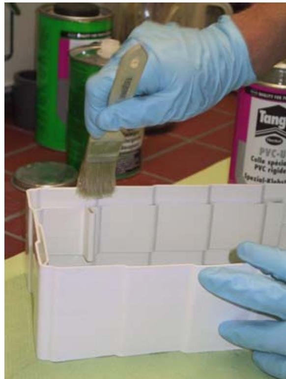
Also glue the surfaces of the coupler with at least 1 1/2in of glue.
