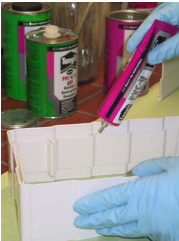
Fill the groove with Tangit PVC-U using it as a sealant.
